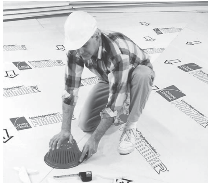
Typical Tapered Roofing Section, 1/8" per foot slope
